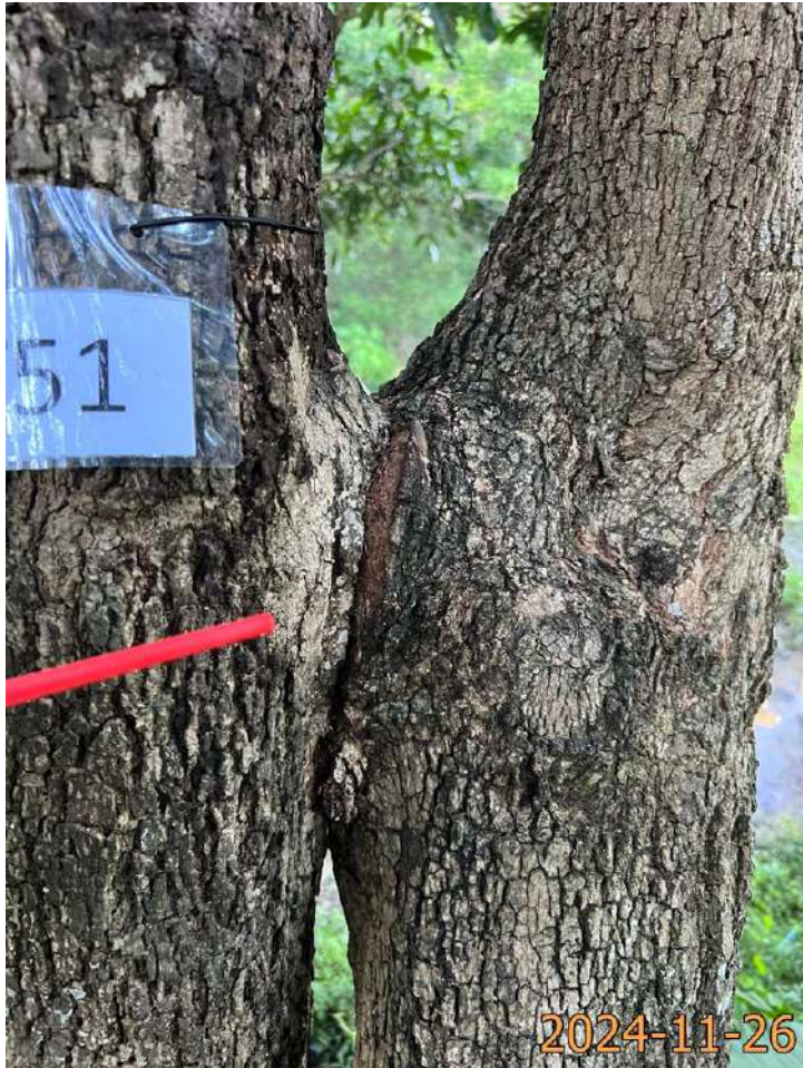
T51 Trunk conflict of co-dominant trunks
